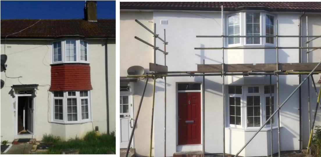
Before and After Insulation Works, dwelling on Flexmere Road, Haringey, London
